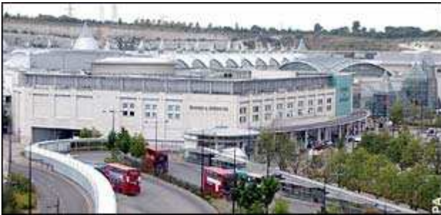
Bluewater Shopping Center, Kent, UK
